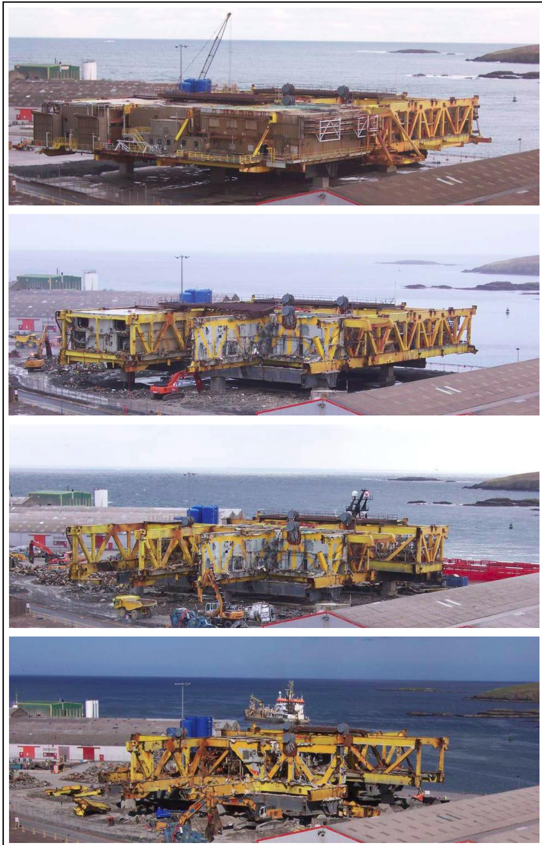
Figure 38: Steps of dismantling topsides (Images courtesy of Veolia Environmental Services)
