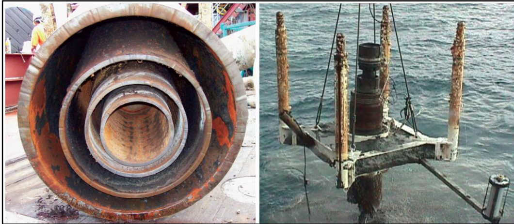
Figure 27: Wellhead sliced by abrasive water jet (left) and wellhead removal (right) (MCGENNIS, 2007)
