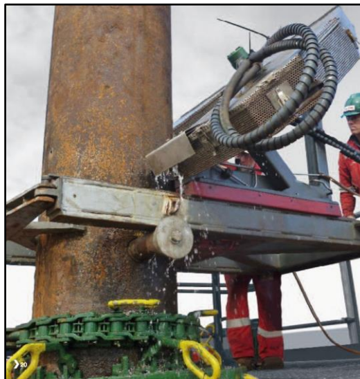
Figure 29: Cutting conductor in segments at topsides (CLAXTON ENGINEERING, 2015)
