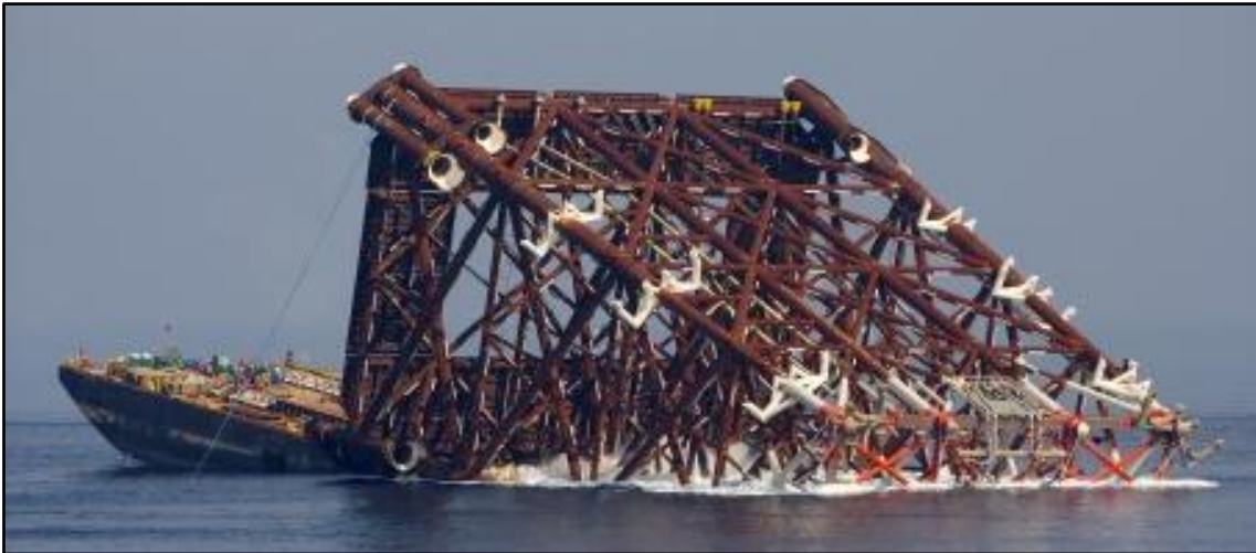
Figure 6: Launching of a jacket off a barge (SUBSEA WORLD NEWS, 2015)
