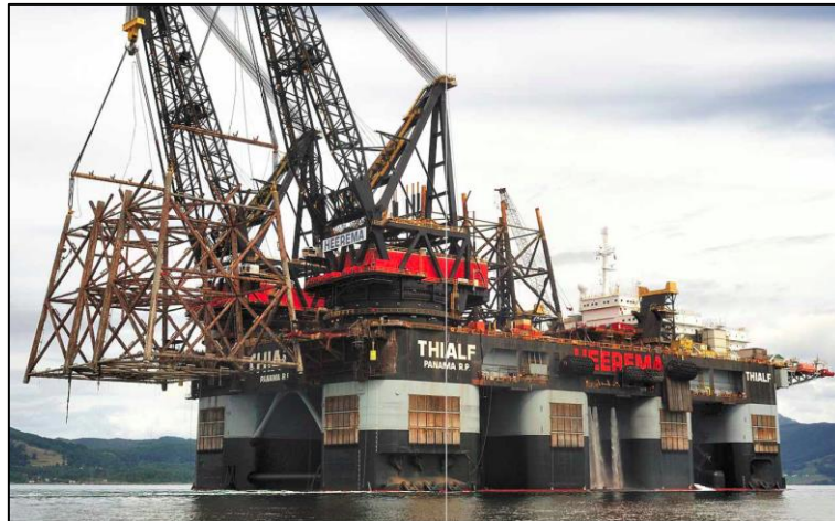
Figure 32: Jacket removal in various steps (DECOM NORTH SEA, 2014)
