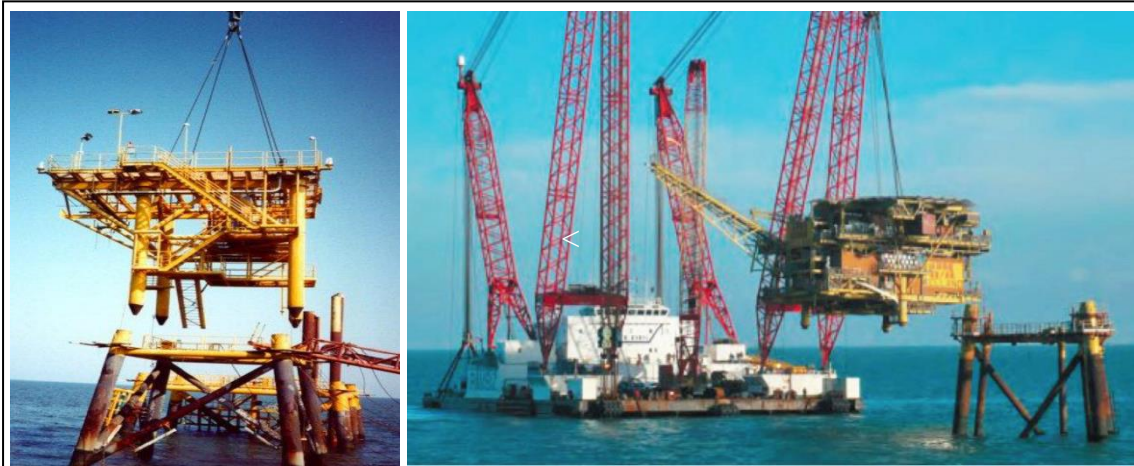
Figure 31: Types of topsides removal, in various steps (left) (BYRD, MILLER, & WIESE, 2014) and single lift with all modules still in place (right) (DECOM NORTH SEA, 2014)
